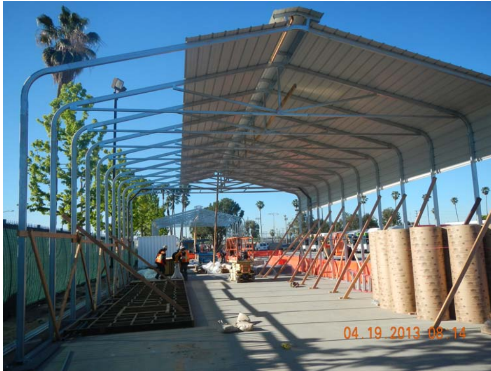
1. Carport canopy structure being erected for temporary fuel islands.
