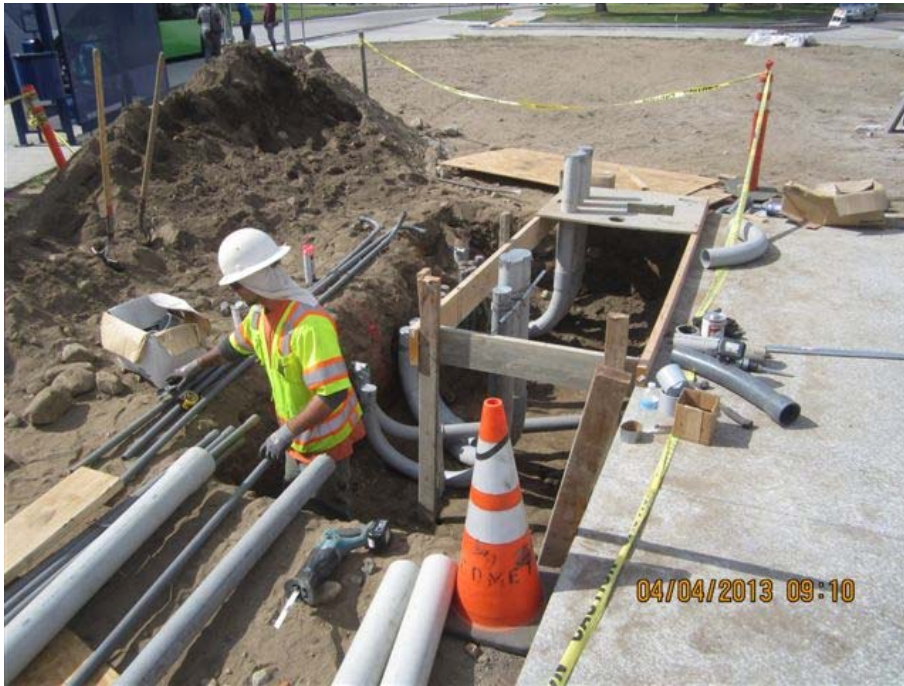
1. Construct Electrical for Equipment Module.
